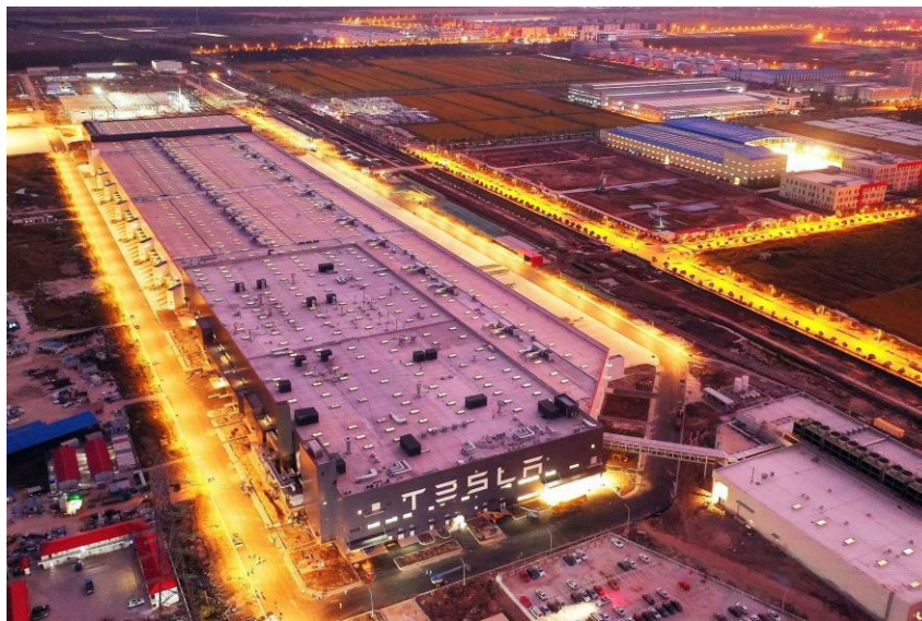
Tesla's Shanghai Gigafactory - built in well under a year.
